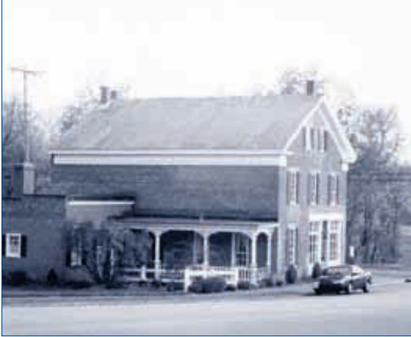
Assistance in nominating properties to the National Register of Historic Places such as Navarre's Loew-Define Grocery Store and Home would help preservation efforts.
