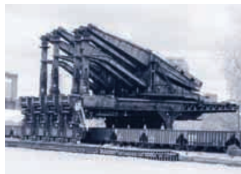
The Hulett Ore Unloaders, standing 100 feet high, revolutionized the U.S. iron and steel industry in the early 1900s.
